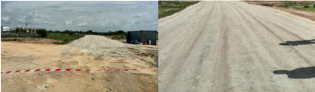
Initial pressure, leveling and rolling of solidified soil
