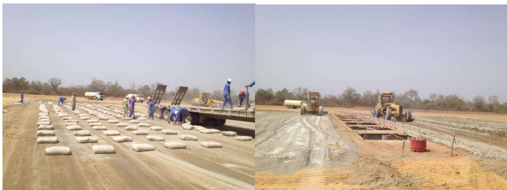
Spreading cement Mechanical mixing
