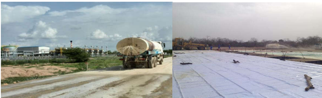
Spraying water and curing agent curing
